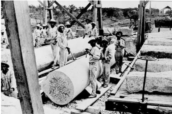
Convict laborers at work on the granite columns for the Texas State Capitol construction, circa 1885. Prints and Photographs Collection, Texas State Library and Archives. http://www.tsl.state.tx.us/exhibits/forever/repression/page5.html
